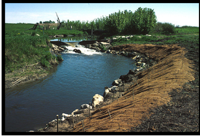
Figure 14. The initial application of a geotextile along a stream bank.
