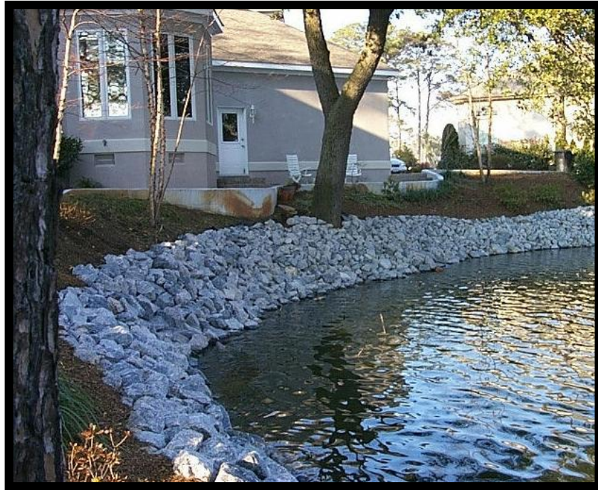
Figure 15. The application of rip-rap along a stream bank to help prevent erosion.
